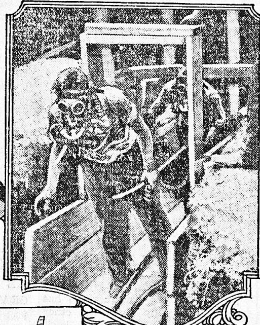
WORKERS IN GAS MASKS AT AN OIL WELL
